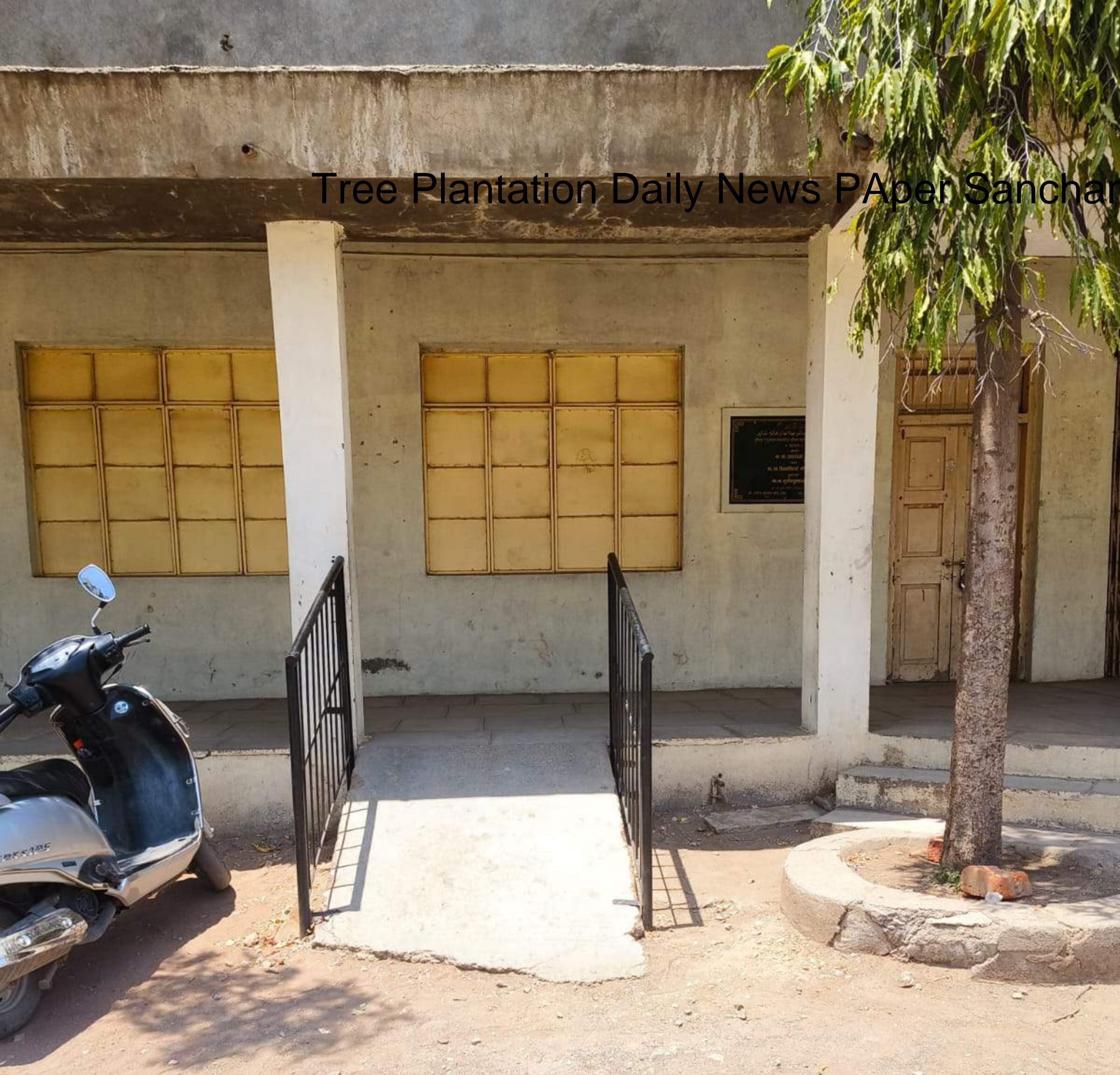
Rail Ramp for Divyangjan
